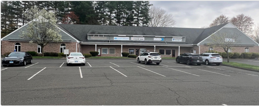
22 Morgan Farms Drive — 1-story brick building (1988), 76 surface parking spaces
